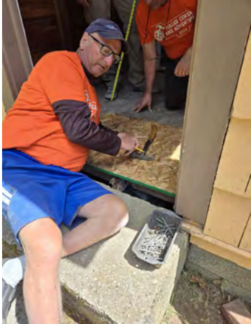
Bicycle Adventurers help to cut out, reinforce, and patch the collapsing porch floor
