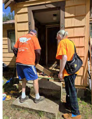
Bicycle Adventurers help to cut out, reinforce, and patch the collapsing porch floor
