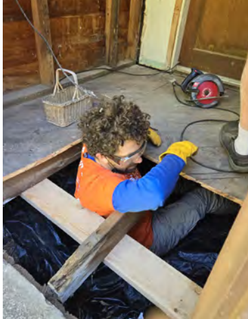
Bicycle Adventurers help to cut out, reinforce, and patch the collapsing porch floor
