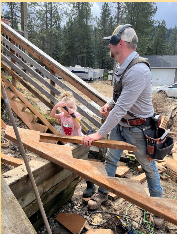
Josh and his daughter work to replace the stairs up to the house. The old stairs were rotten and dangerous
