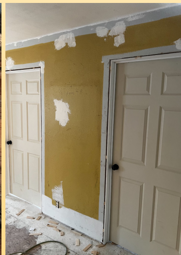
New interior doors and walls prepped for paint
