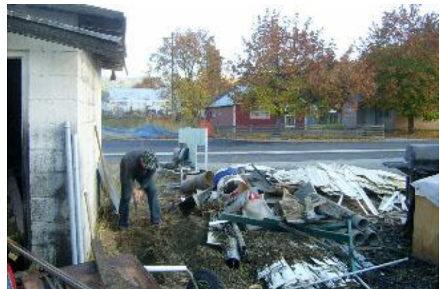
Tully Fedilley helps by extending the drain ditch. Later others including Rick Wood & Verne filled it with gravel. We are working on creating covered space for all the materials stacked in the rear of the ReUse Store.
