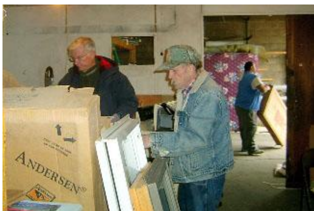
Ed Vang, Bob Larson, and Mike Humphrey sort and move windows, making more room in the display area. This also created room for the workers to have access for the equipment to blow more insulation. Photos by Judy
