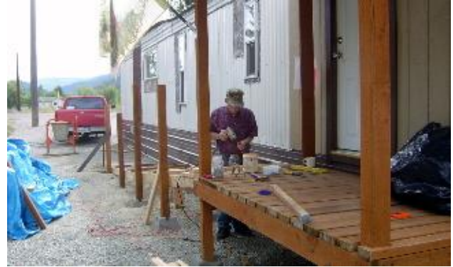
Bob Larson constructs a "Greater Blessings" handicap ramp in Osburn.
