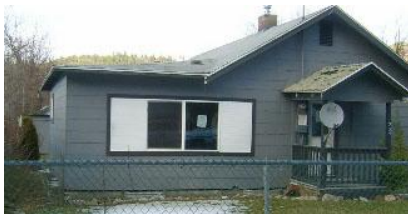
HUD House in Smeltonville
