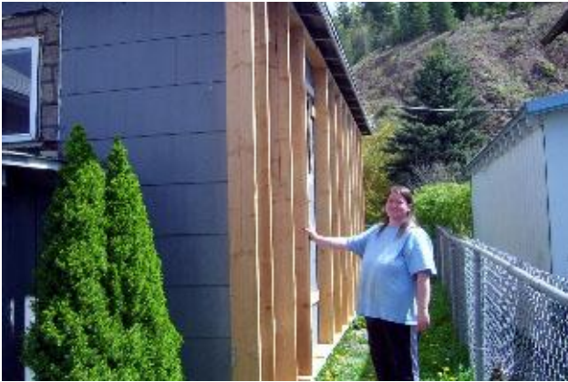
Darnell Kriedeman shows how a new insulated outer wall will help make her home "green" by conserving heat energy. Our visiting work groups, the RV Builders, Fuller Center Bike Adventurers, and kids from Shoshone Base Camp will help finish insulating and siding these walls.
