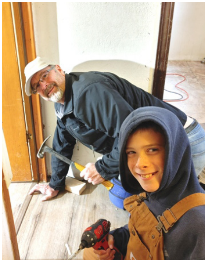
Ken Morris and Jedidiah Braunstein install flooring in the Osburn trailer
