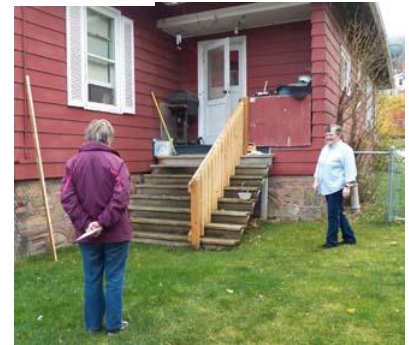
Mary Kay Hanson, at right, shows the railing installed as a Greater Blessings project at her home.
