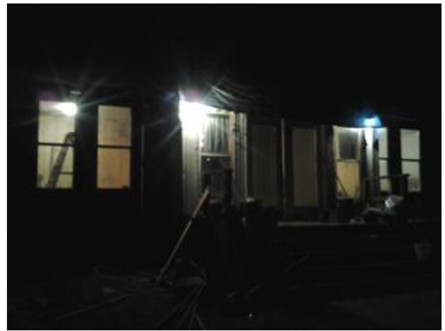
Light glows through the new windows in the bedrooms on both sides of the Mace's front door. They were installed by Greater Blessings volunteers, Rick Gilbert, Rick Wood & Mike Humphrey and Mace kids. Photo by Christina
