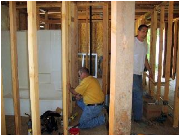
Several SBC volunteers helped Verne pull wires. Photo by Mike Humphrey
