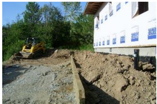
John Hopper did the back fill against the foundation along the Lake home.
